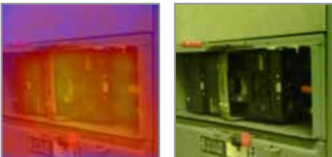
Normal operating temperature on mission critical breaker
