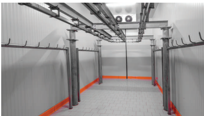
Cold Room and Storage
