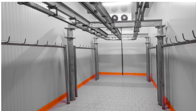
Cold Room and Storage
