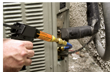
Step 3: Inject, then discard empty cartridge.
