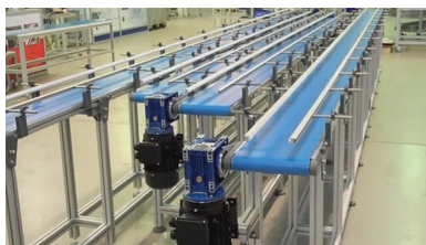
Figure 2.3 Monitoring vibration and temperature in conveyors.
