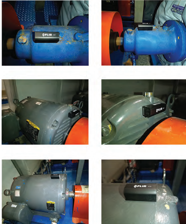
Figure 6.2 SV87 Sensors shown mounted on machinery.
