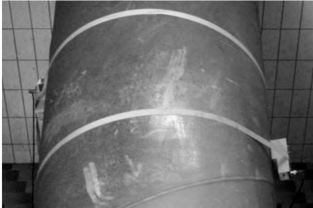
FIGURE 33: Z-mode installation with fabric-reinforced tensioning tapes for large pipe diameters
