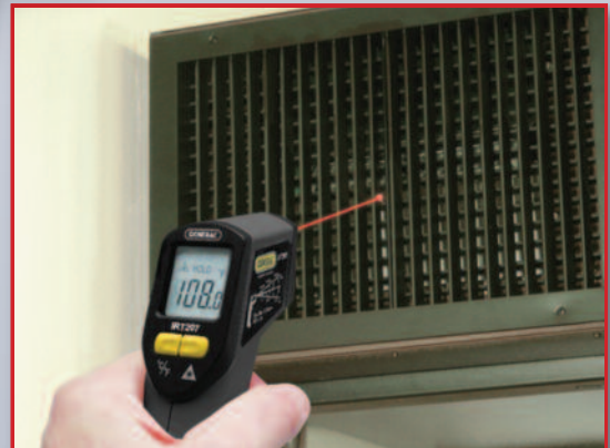
Performance-testing a new A/C system
