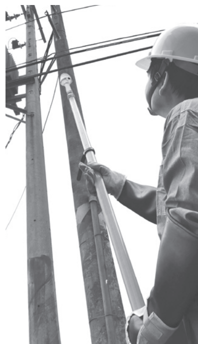
Fig. 3: Voltage detection for overhead lines
