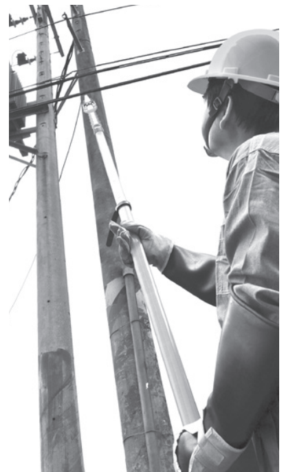
Fig. 3: Voltage detection for overhead lines
