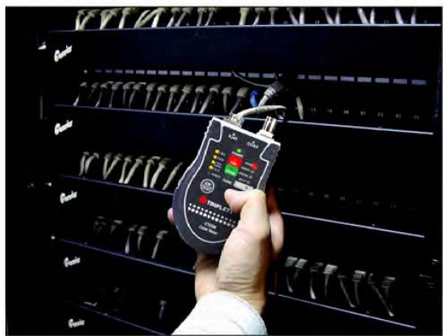
Confirm continuity and fault type
