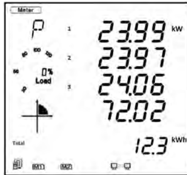
Figure 3-7 - Three-Phase Power Page
