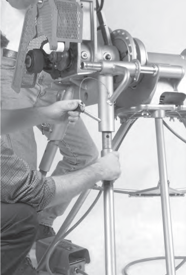
Figure 5 – Installing Legs Into the Groover Base
