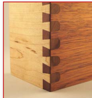
Cuts Through Joints
