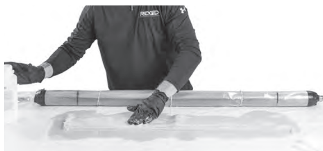
Figure 28 – Wetting Out The Patch Off The Packer
