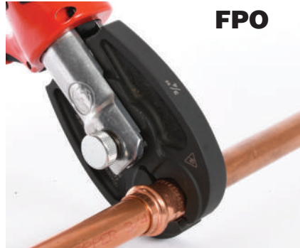
Figure 9 – Placing Jaws Around Fitting
