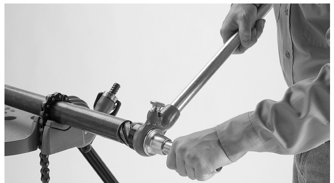
Figure 4 – Reaming End Of Pipe
