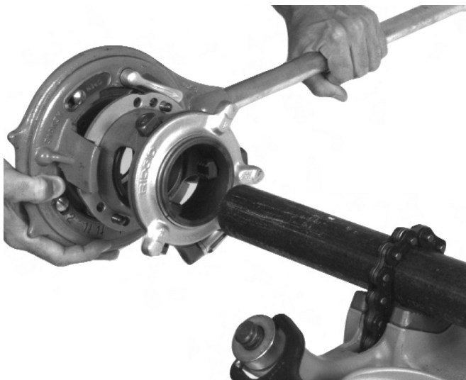
Figure 5 – Sliding Threader Onto Pipe
