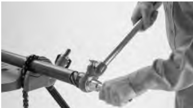
Figure 2 – Reaming End of Pipe
