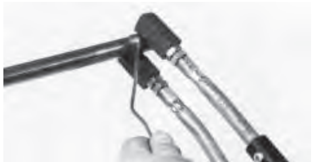
Figure 6 – Soldering Joint
