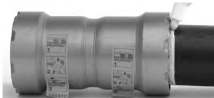
Figure 7 – Marking the Pipe After Fully Inserting Pipe
