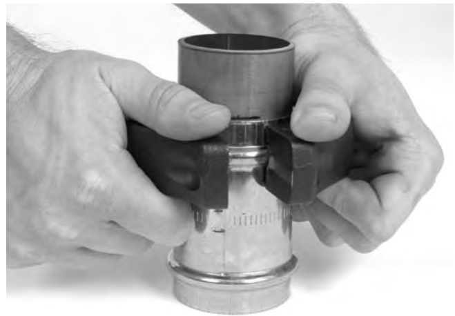
Figure 8 – Installing Press Ring Onto Fitting
