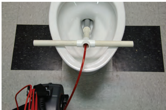
Figure 23 – Using a PVC Guide Tube
