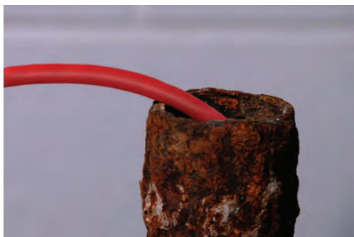
Figure 16 – Avoid Pulling at Sharp Angles
