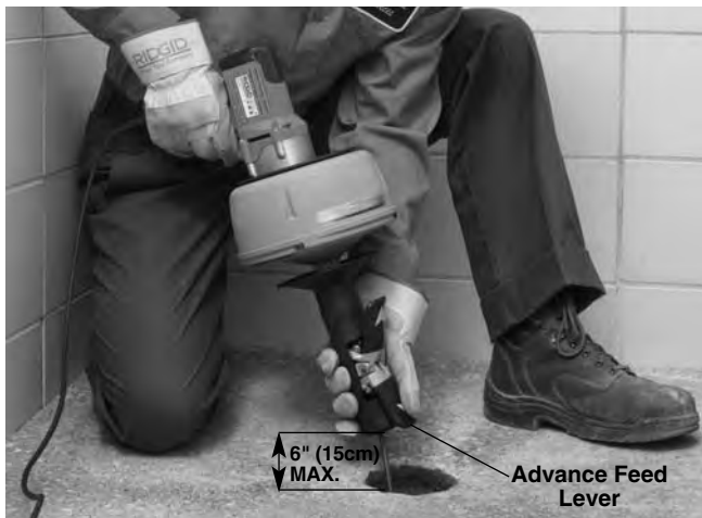
Figure 10 – Feeding Cable With AUTOFEED
