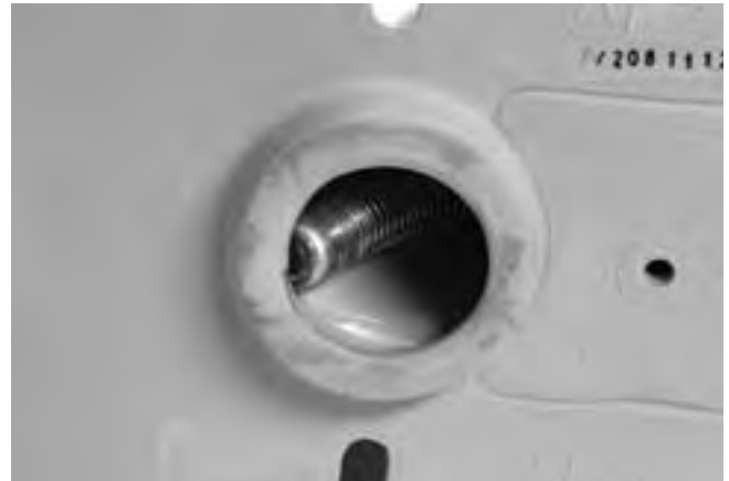
Figure 20 – Camera Head Blocked in Turn
