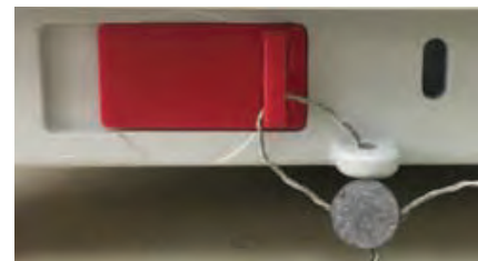
Locked with Wire Seal
