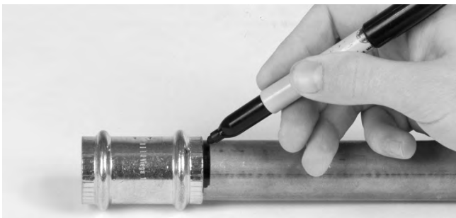
Figure 8 – Marking the Tubing After Fully Inserting Tube
