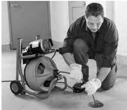
Figure 13 – In Operating Position, Manually Feeding Cable
