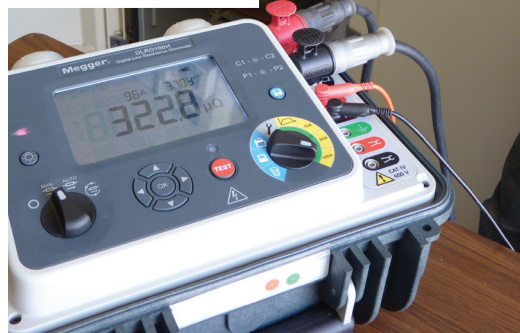
DLRO100H testing rack-mounted, 3-phase circuit breakers
