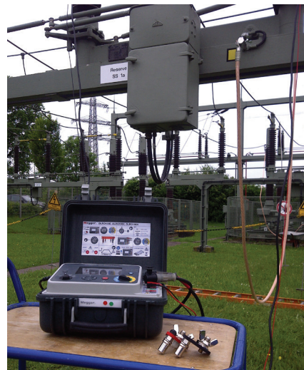
DLRO100 testing circuit breaker
