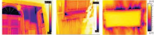
Insulation - Energy Loss, Home Inspection, and HVAC
