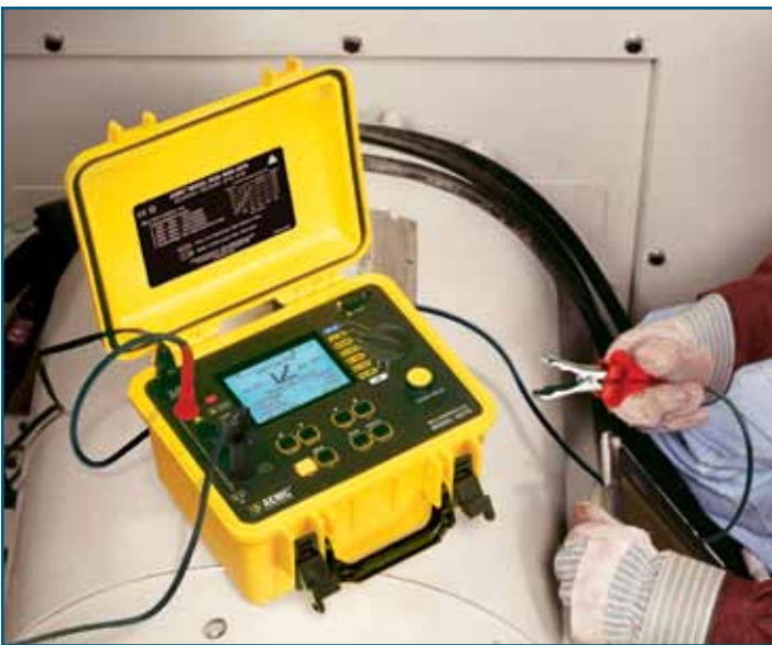
Model 5060 performing insulation test on a generator.
