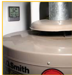
Monitoring Dew Point levels in a Basement for potential mold growth.
