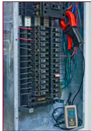
L101 recording branch circuit current.
